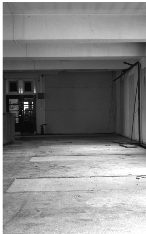
FHO after demolition (July 2001, photograph: S.A. Harris)
