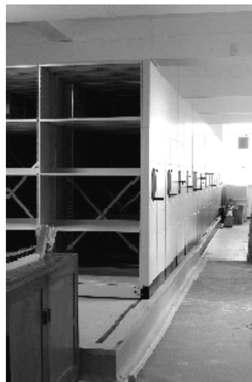
Refurbishment work in progress in FHO (January 2002, photograph: J. Baker)
