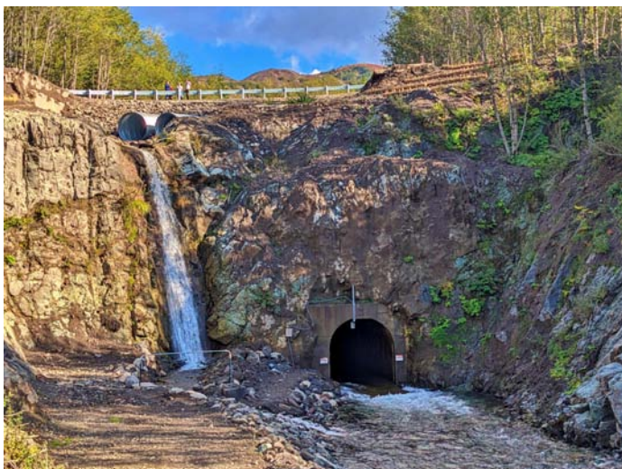
Spirit Lake's level is currently managed by this tunnel, which needs significant repairs to maintain its reliability. PHOTO: SUSAN SAUL
