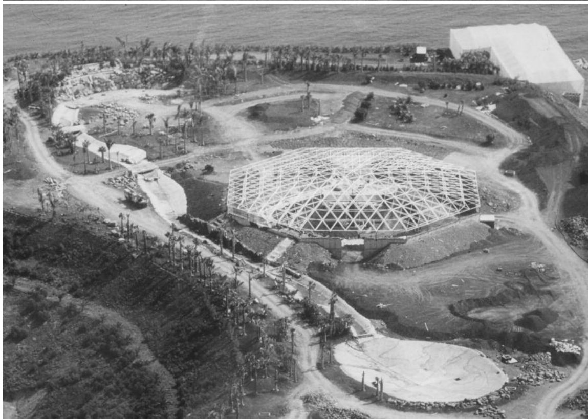
3 (top). November, 1997. River beds are built. 4 (bottom). Aerial photographs of the top of the hill taken in late 1998.
