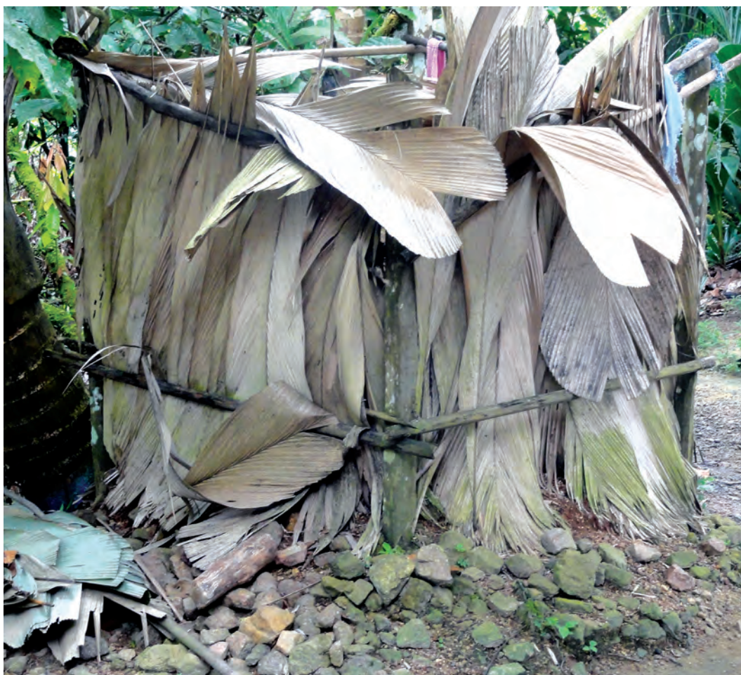
7. Privy constructed with Sclerosperma profiziana leaf blades near Ankasa Conservation Area (Western region).
