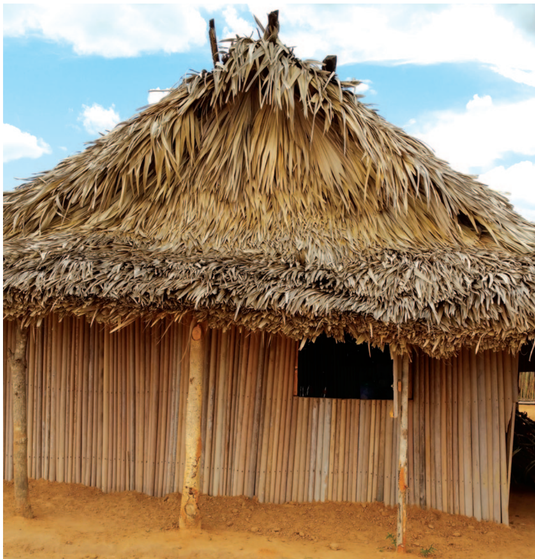
1. A Sakalava house thatched with the leaves of Hyphaene coriacea and with walls made from Raphia farinifera petioles.
