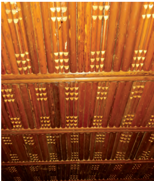
8. Detail of a ceiling made with raphia petioles (bamboo), Bamendjinda, 2017. Photo by Ariane Cosiaux.
