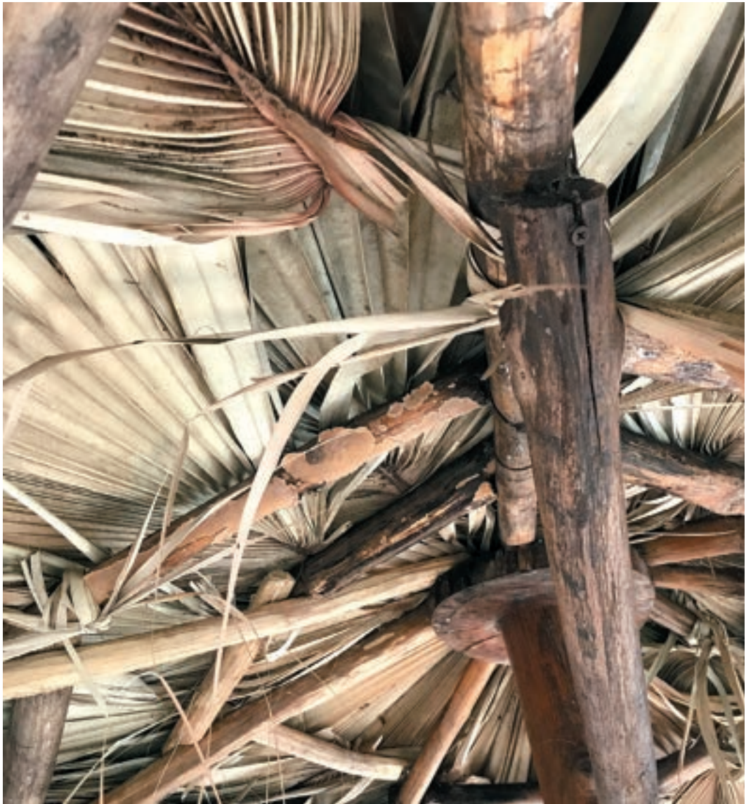
3. Detail of a palmiche -roofed rancho . If well-made, these structures are waterproof and can last for several years.
