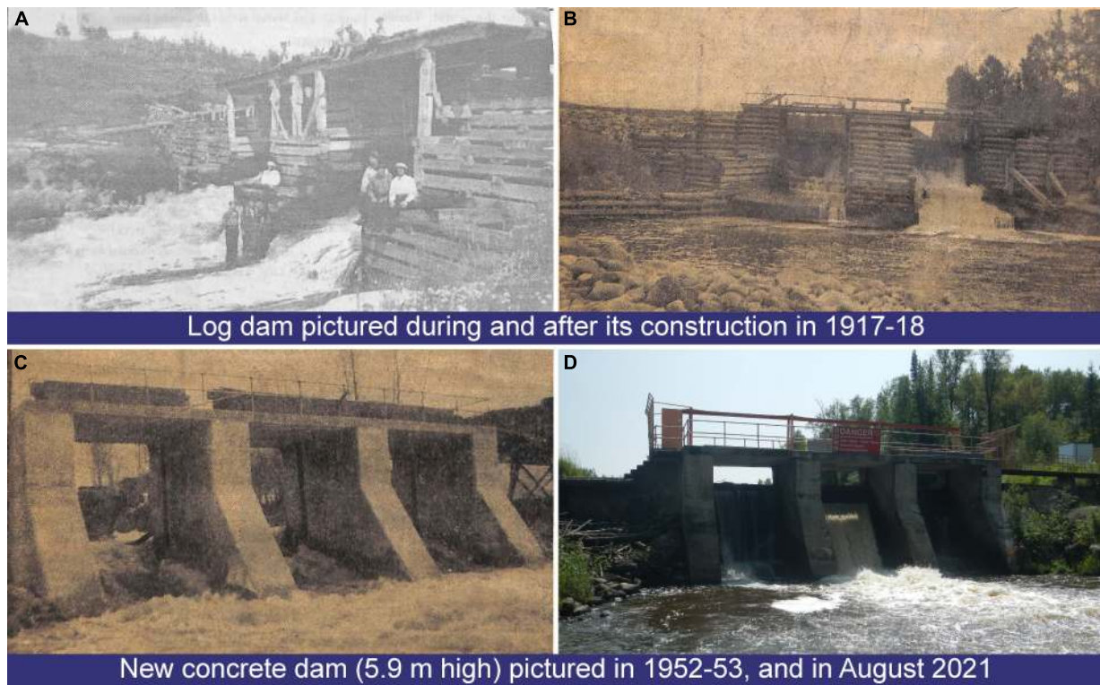
FIGURE 2 | The old and the new on Driftwood River at Monteith. First log dam (A,B) and second concrete dam (C) in the years of their construction as compared to today structure (D). Historical photos (B,C) by Mrs. C. Clifford were published in an unknown local newspaper on May 6, 1953. All historical photos retrieved from the digitalized archives of the Monteith Women Institute Tweedsmuir Community History, a courtesy of the Federated Women's Institutes of Ontario (FWIO; https://collections.fwio.on.ca ). Photo in August 2021 by AFN.
