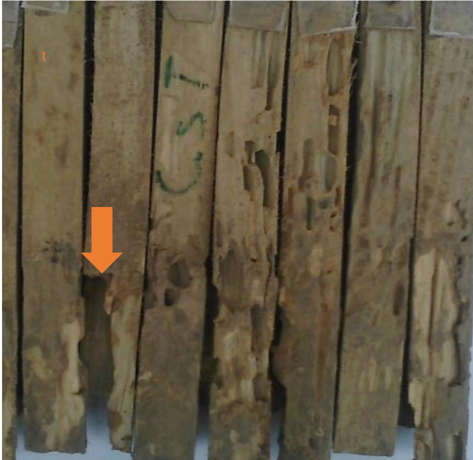
Plate 3.6: Coppiced P. erinaceus sapwood: Top position after 12 months of field exposure (Arrow shows severe termite attack).
