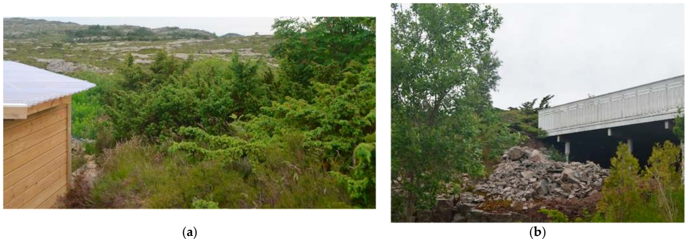
Figure 18. Vegetation dominated by junipers close to wooden constructions 500 m downwind from the jumped fire: (a) Junipers close to, and Calluna touching, a garage; (b) Junipers touching a south-facing wooden balcony.
