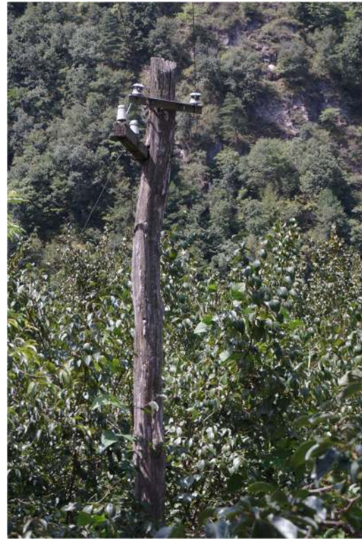
Fig. 22 Up until recently electricity poles were made of Castanea trunks
