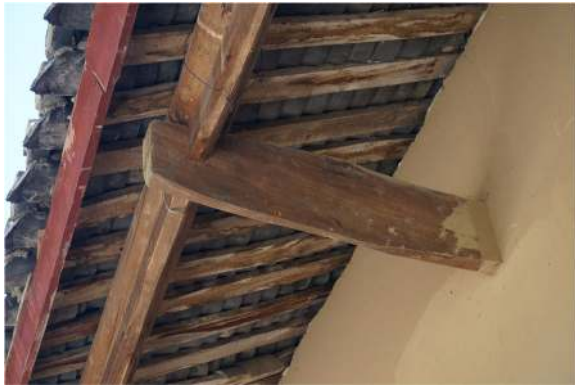
Fig. 16 Boards supporting tiles are often made of Toxicodendron vernicifluum wood
