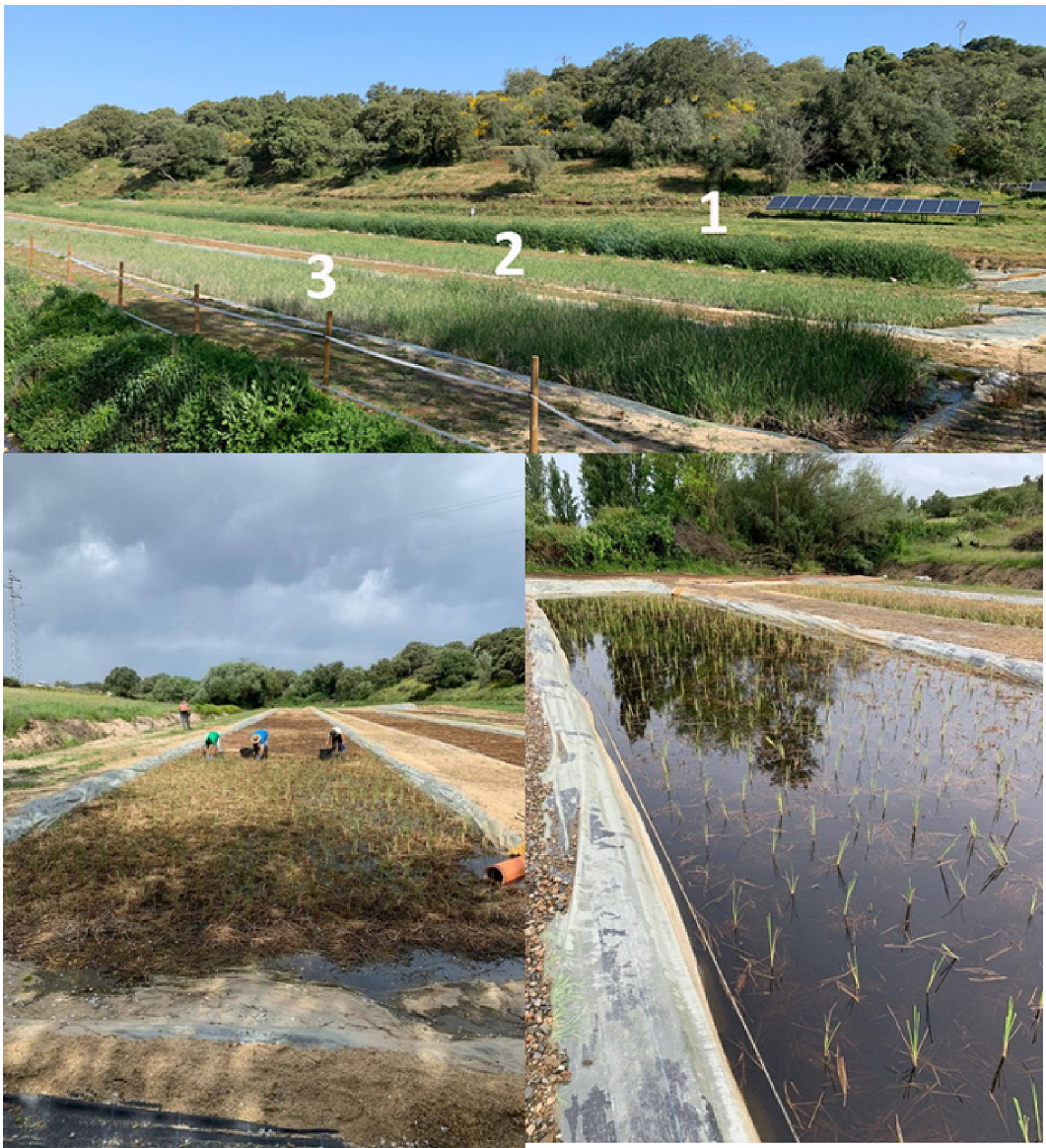
Fig. 2. Different stages in the process of construction, maturation and exploitation of the Typha domingensis floating constructed wetland (numbers indicate the channels). Photographs courtesy of Mr. César Martín (Viveros La Dehesa S.L.).
