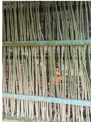
Wall with MS sections
