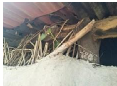
Portion of wall kept open for ventilation
