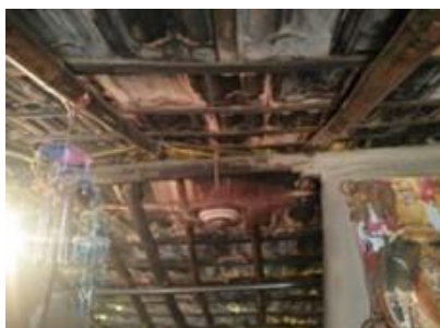
Mangalore Tiles Roofing
