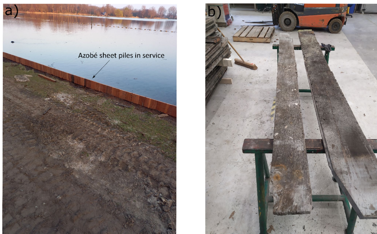
Fig. 1 Full size azobé sheet piles (a) in service at Delftse hout, Delft, The Netherlands; (b) pulled out after 57 years of service from Medemblik, the Netherlands
