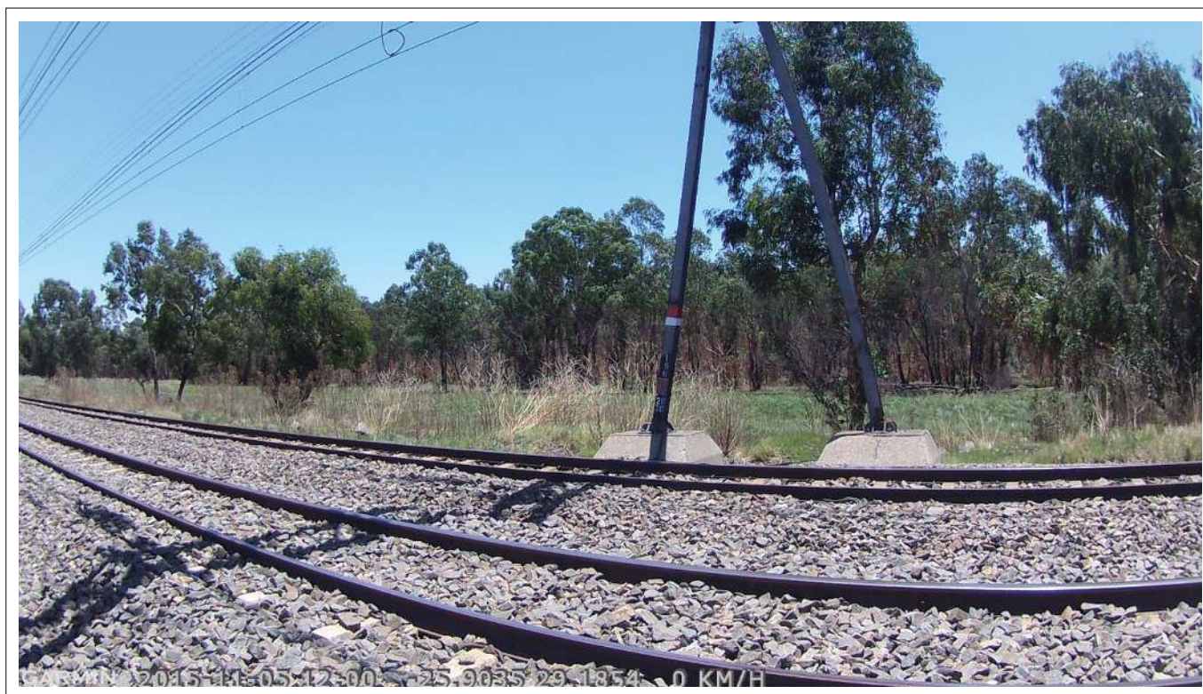
FIGURE 5: Eucalyptus species that appear to be planted but poor control measures have resulted in some plants growing close to the railway infrastructures.
