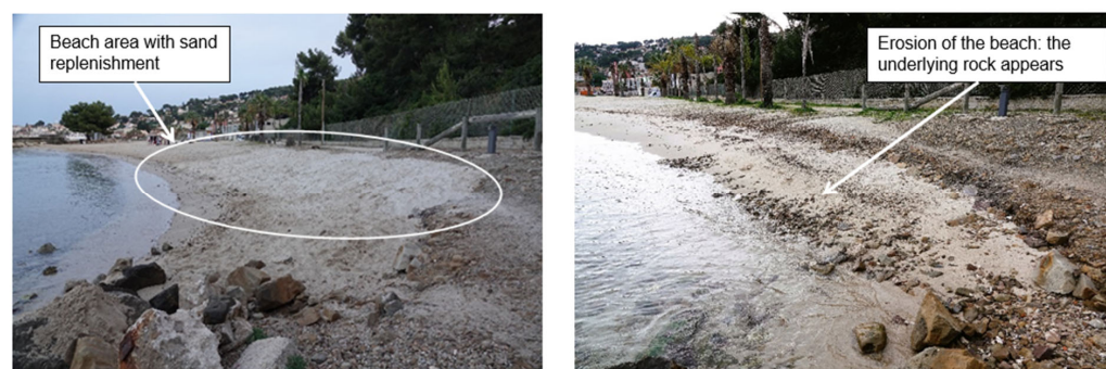
Figure 8. The La Vieille beach is annually replenished with quarry sand. (left) Late June 2023, just after replenishment. (right) Late summer (September) 2023. Photos © Dominique Calmet.
